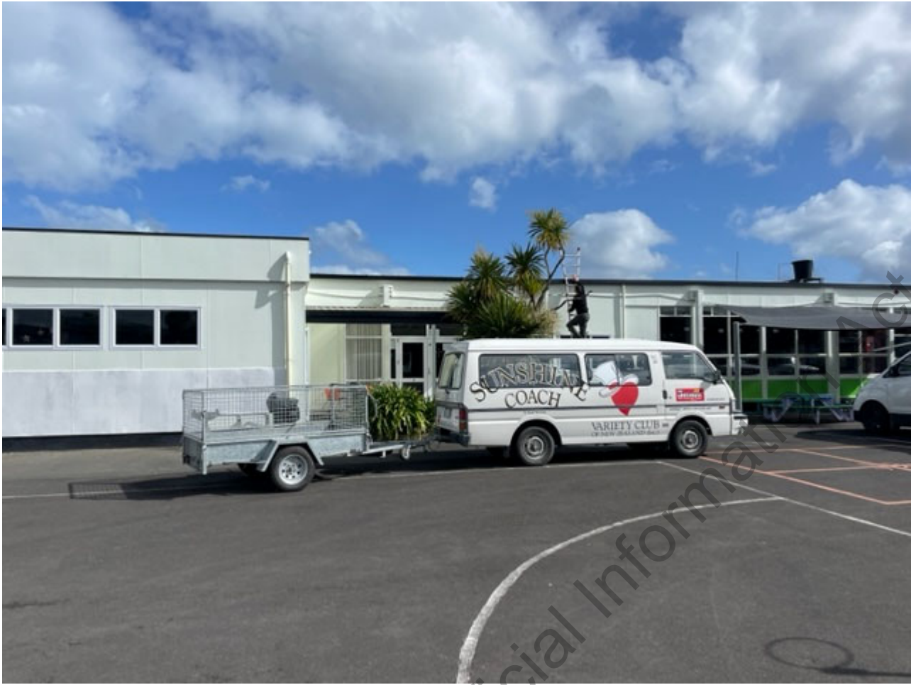
Block E Ceiling issues
