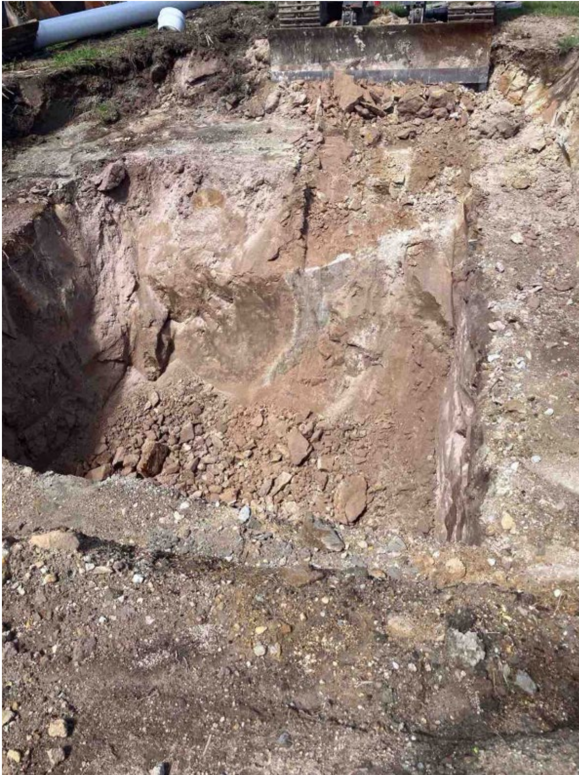
Wet Well Excavation in Progress
