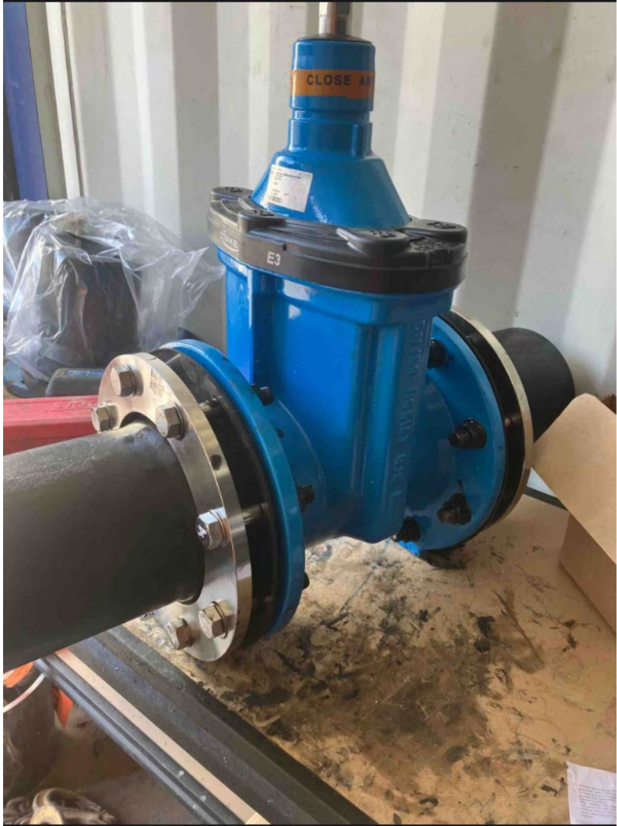
Valves being bolted together
