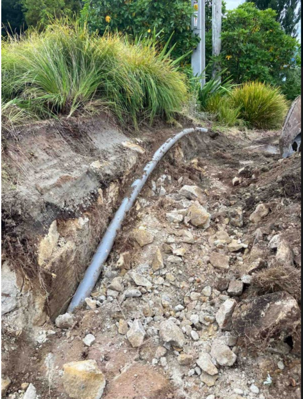
Unknown Chorus discovered whilst removing earth bund for pumpstation
