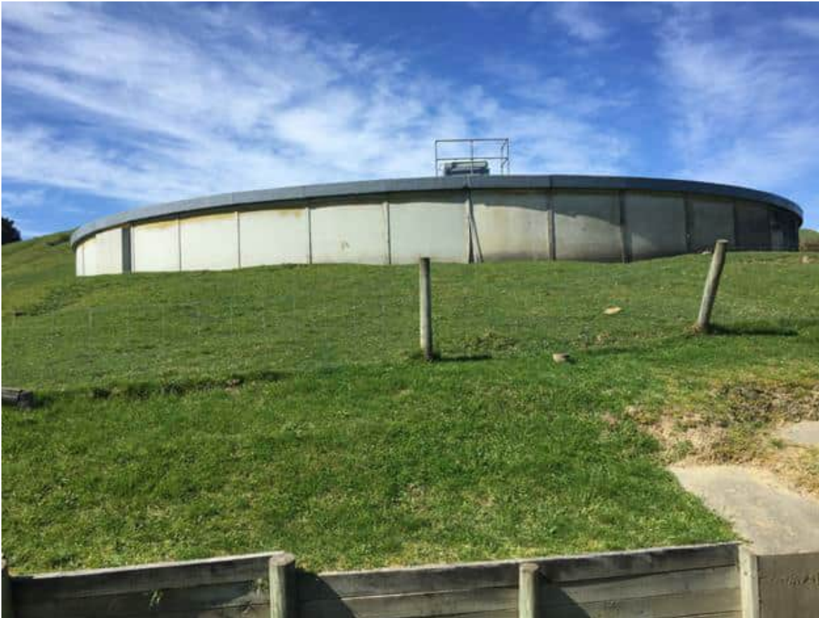
Figure 2-24: Example of reservoir partially built into hill – Sutherlands 1 Reservoir
