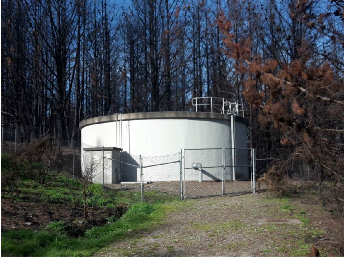
Figure 2-23: Example of above-ground reservoir – Worsleys 2 reservoir
