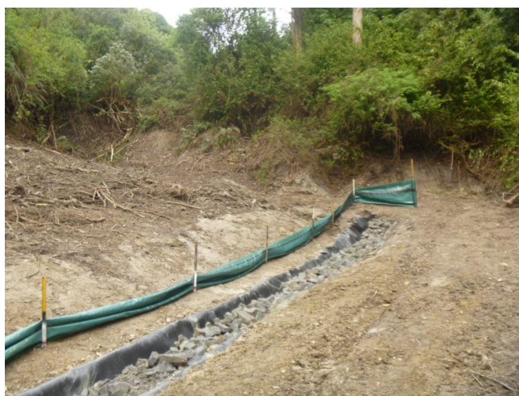
Figure 7:1 Scour protection of interceptor drains above Wingatui Tunnel MSL
