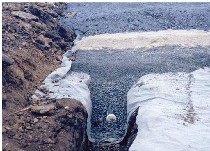
Figure 7:13 Example subsurface drain (photo courtesy of Maccaferri)
