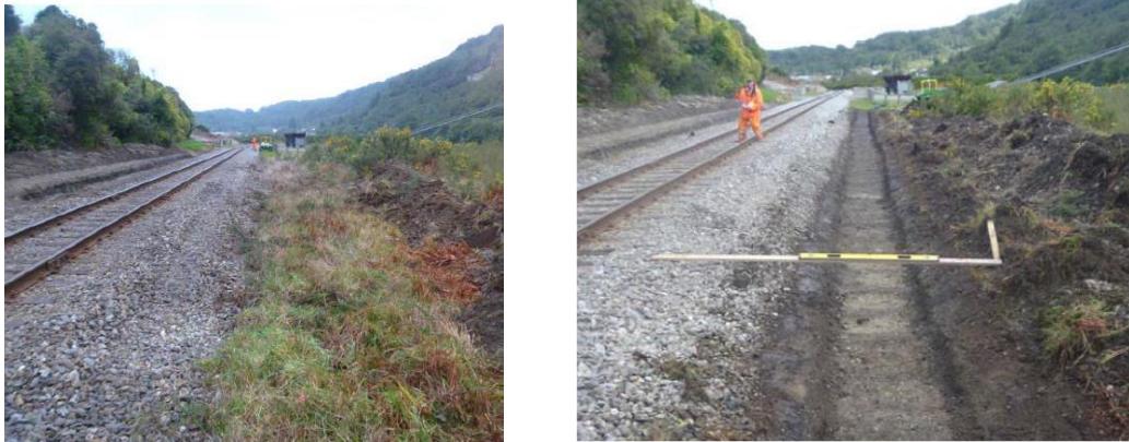
Figure 7:8 Cess drains at 198km Midland Line before and after upgrade work
