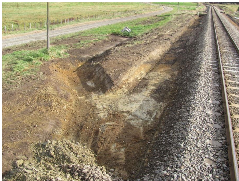
Figure 7:11 Mitre drain at 30.8km MNPL
