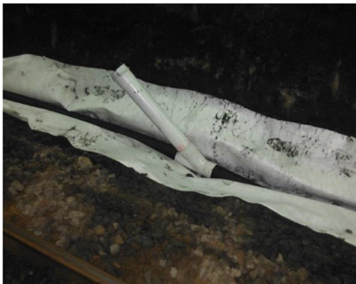
Figure 7:18 Y' Connection of cleaning eye to Nexusflo pipe, Caversham Tunnel MSL
