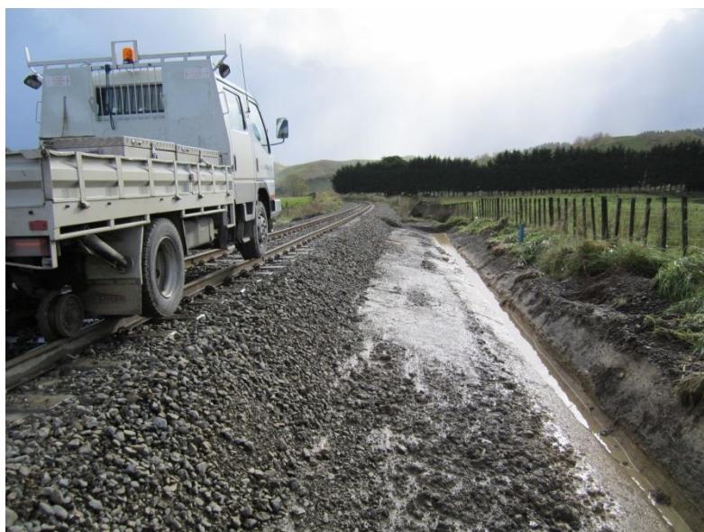
Figure 7:4 Cross fall of formation cess/shoulder, 31km MNPL, to assist ballast drainage
