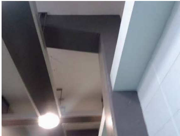
Photo 15: End of original concrete frame at ground at the corridor side
