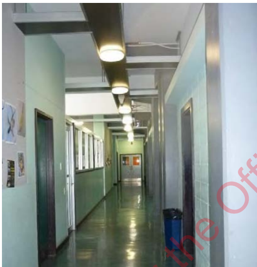
Photo 11: Corridor at ground floor level showing the addition/extension
