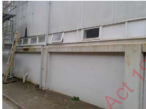
Photo 10: Detail of east elevation with the original precast panels at ground floor level
