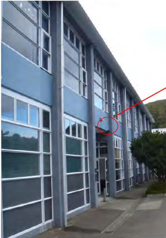
Photo 5: Mid-section of West elevation
