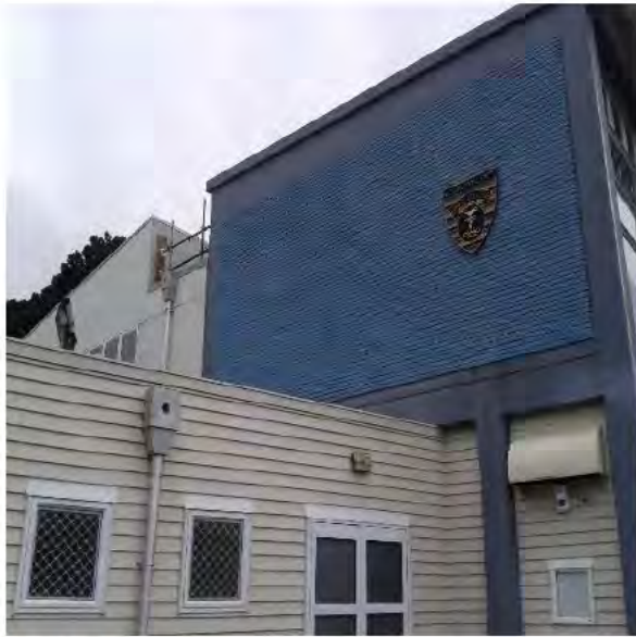
Photo 1: North elevation showing veneer on top floor infill panel
