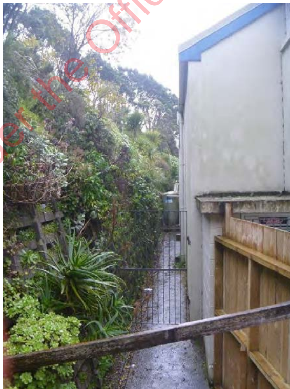
Rear of building (South Elevation)
