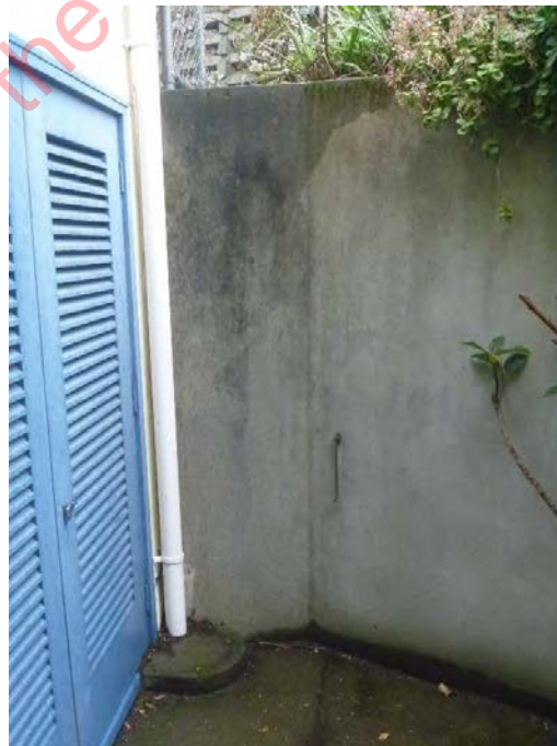
Figure 2: Reinforced concrete retaining wall
