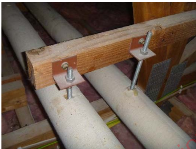
Figure 6: Pipe hangers
