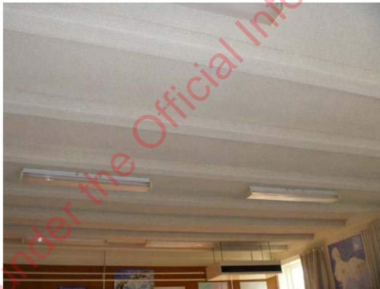
Ground Floor Classroom
