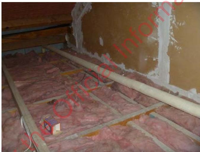
Figure 7: Pipe support
