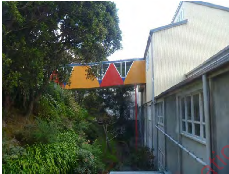
South Elevation and Bridge
