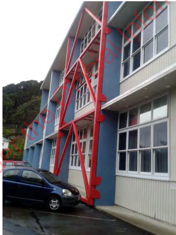
Front Elevation Braced Frame
