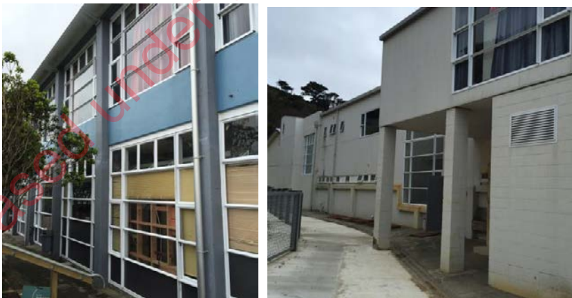
Pictures 1 and 2 - External view of the front and rear of Block 4
