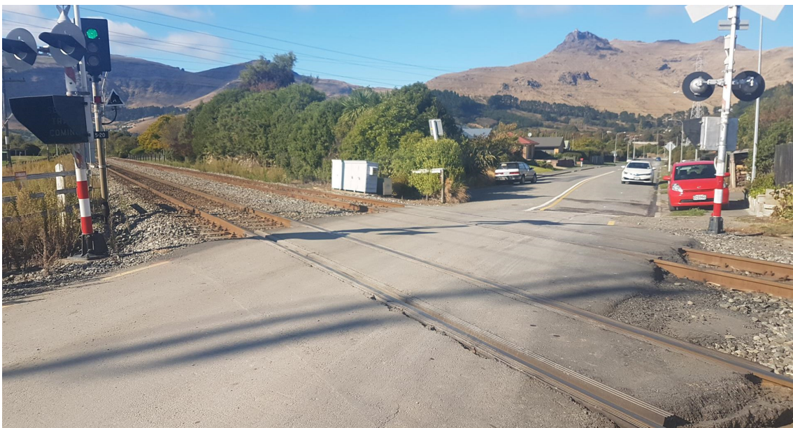
Figure 3-2: Existing Crossing - Looking South
