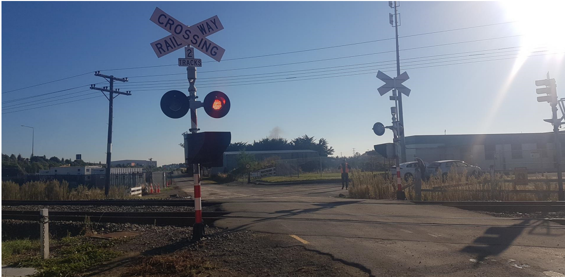
Figure 3-1: Existing Crossing - Looking North
