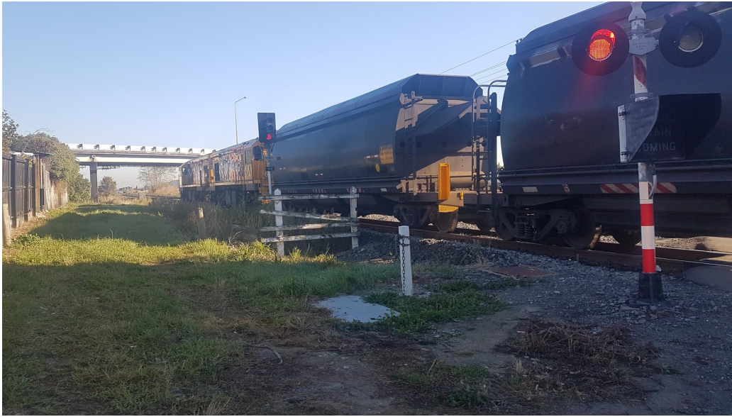
Figure 3-7: Existing service boxes
