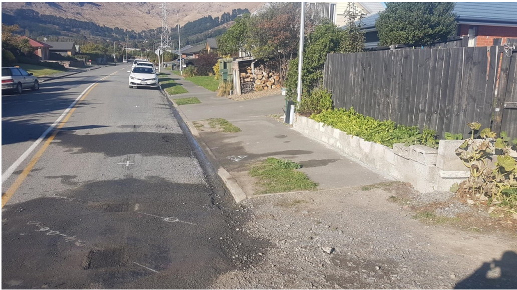
Figure 3-8: Driveways close to LX
