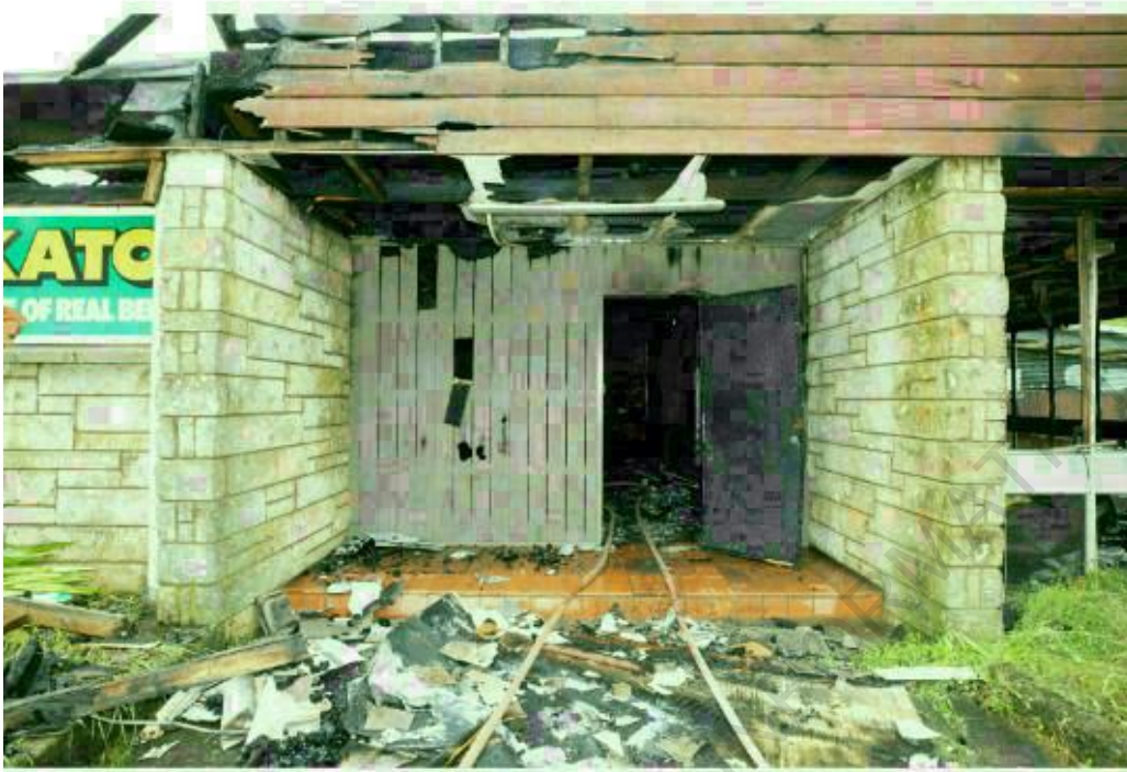
Photo 24: Northeast entrance to tavern. (Photo courtesy of Police).
