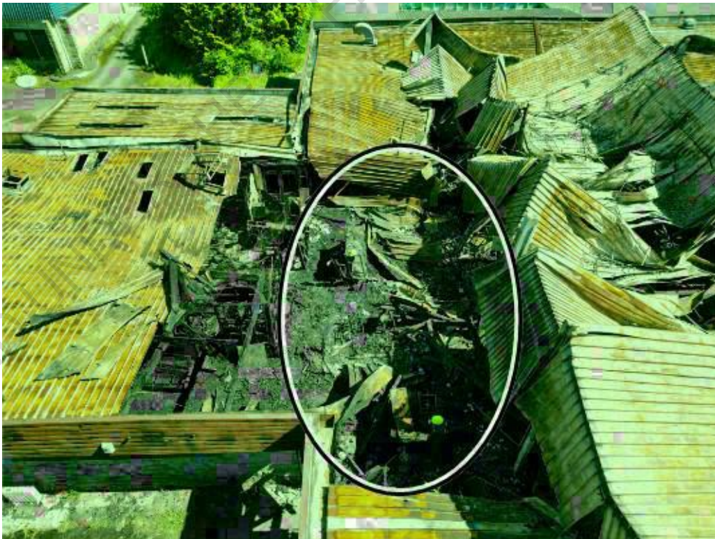
Photo 38: Area of origin after the removal of the roofing iron. (Photo courtesy of Corporate Risks).
