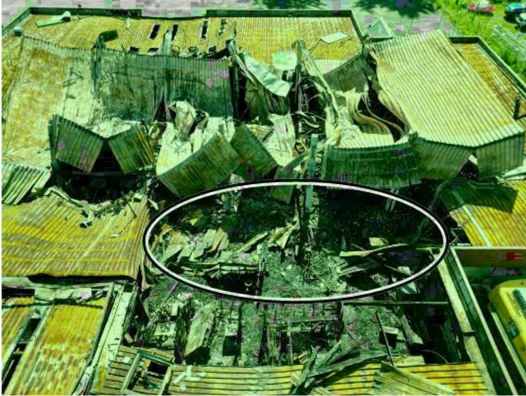
Photo 38: Area of origin after the removal of the roofing iron. (Photo courtesy of Corporate Risks).
