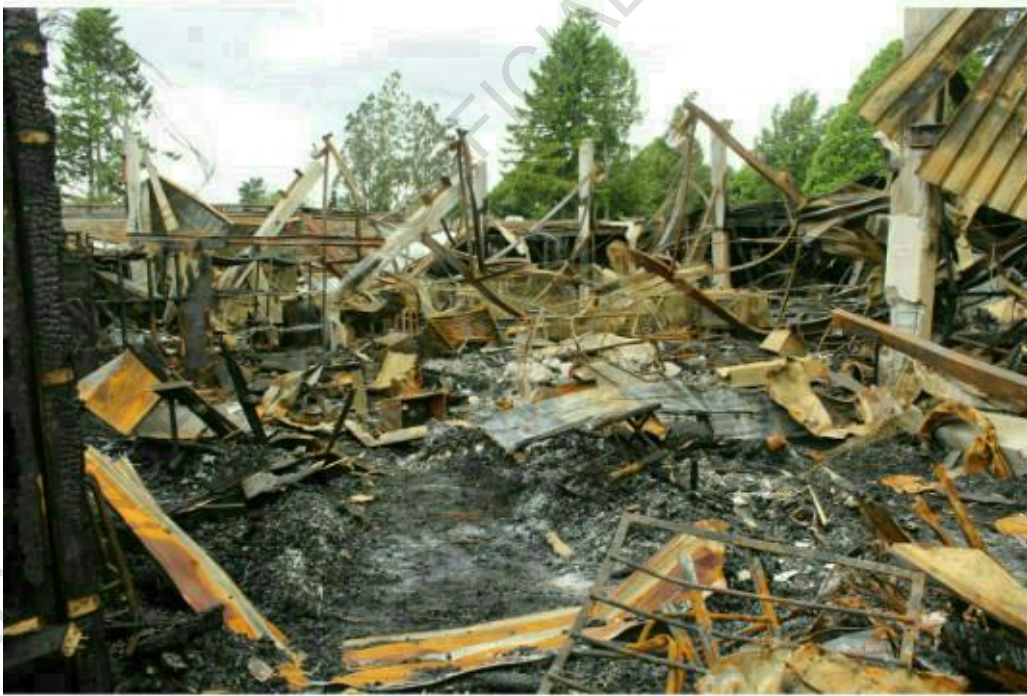
Photo 34: Interior of tavern after the removal of iron and debris.
