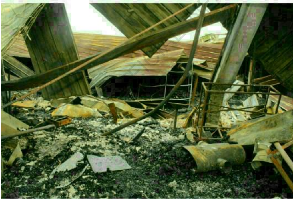
Photo 29: Area in front of the west side tavern bar.
