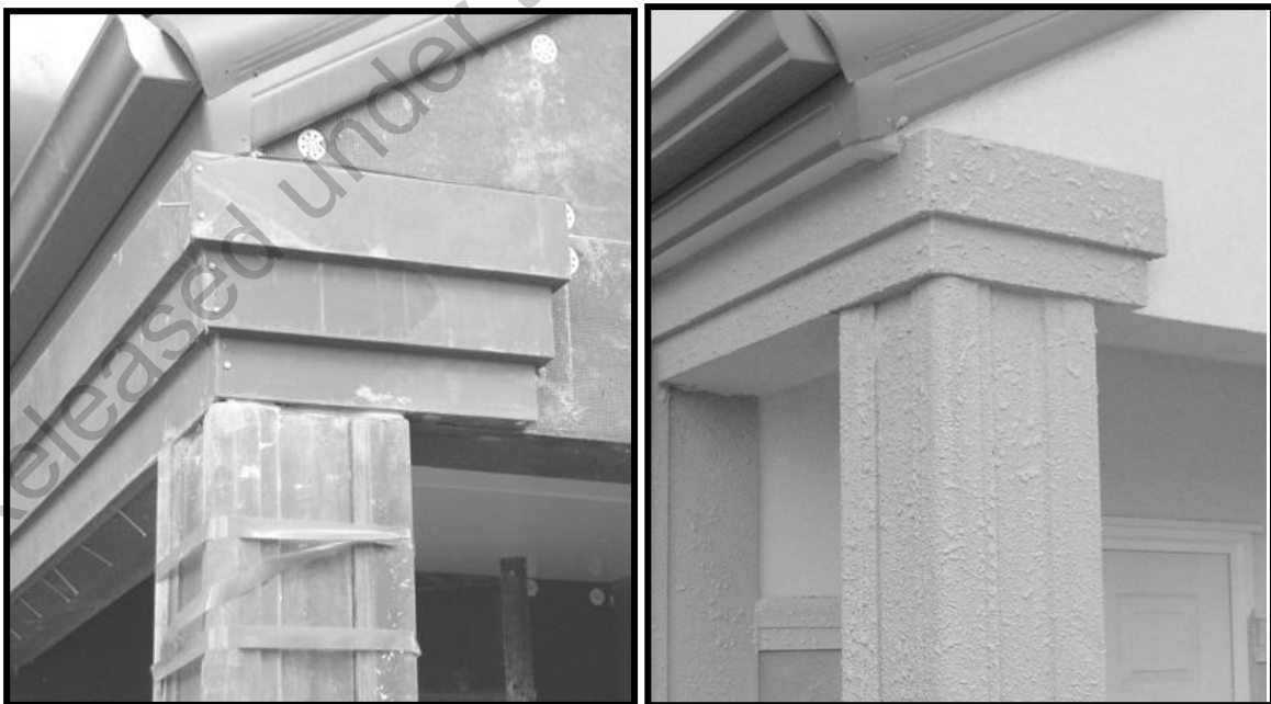
Fig 6.5 Polystyrene features pre and post finishing
