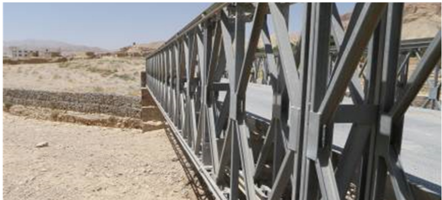
A bridge in Sayghan district that was repaired using CERP funds
