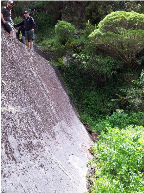
Photo 21: Dam downstream face and left abutment contact.
