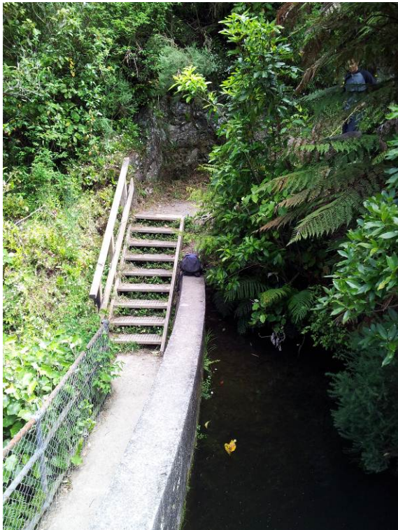
Photo 28: Dam contact with right abutment
