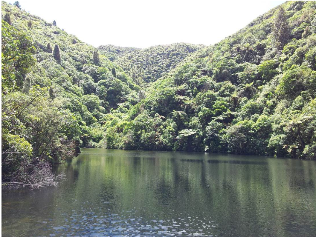
Photo 24: Birchville Dam reservoir
