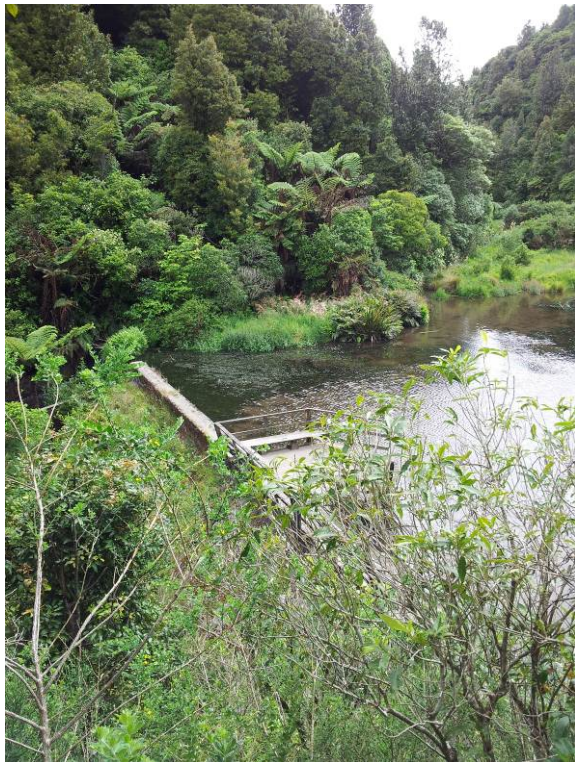
Photo 1: Korokoro Dam looking upstream to head of reservoir. Spillway entrance in middle left.
