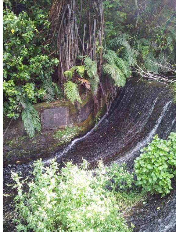
Photo 4: Spillway crest and right abutment contact.
