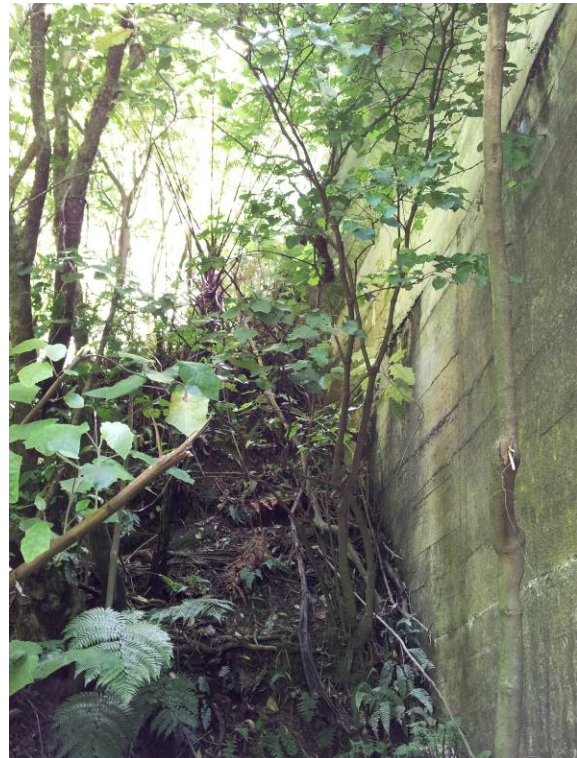
Photo 29: Downstream contact with right abutment.
