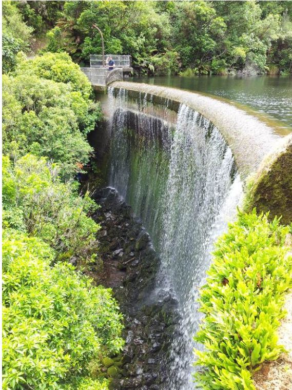
Photo 26: Birchville Dam spillway crest and toe from left abutment.
