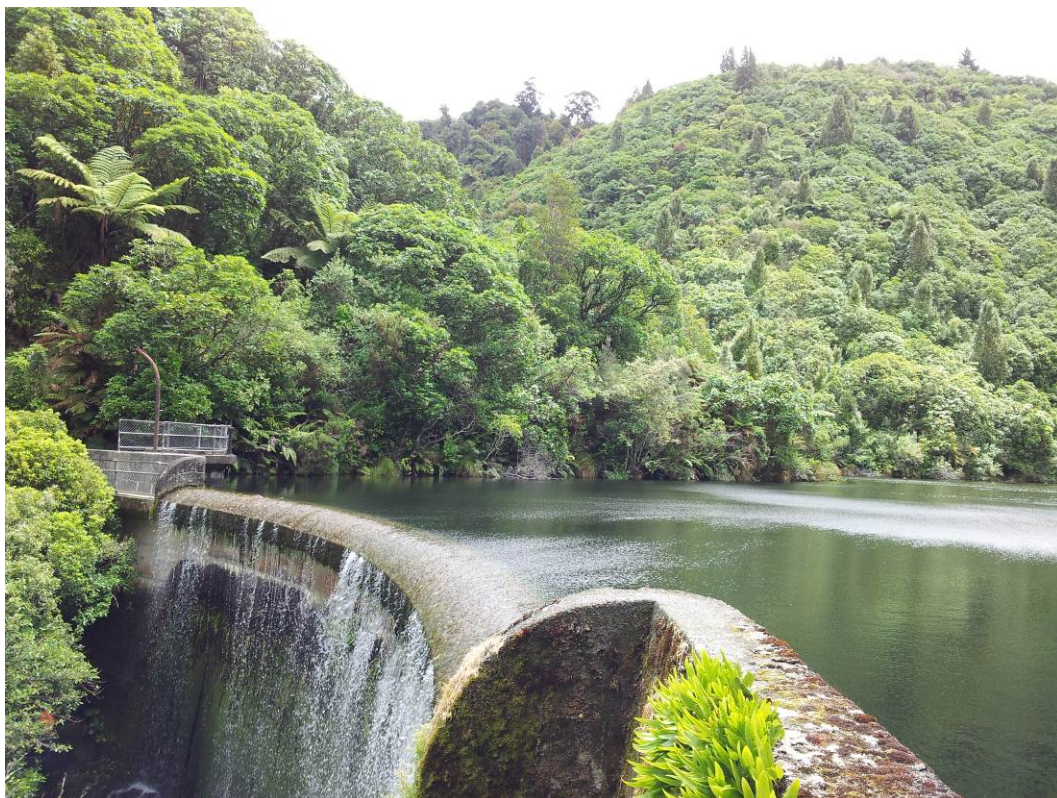
Photo 25: Birchville Dam spillway crest and right bank reservoir
