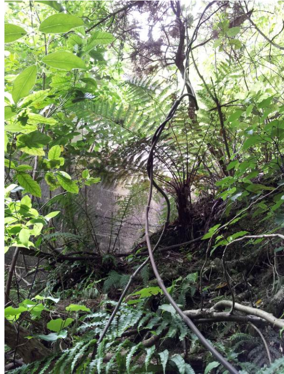
Photo 31: Downstream contact with left abutment.
