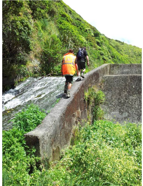
Photo 20: Spillway chute and chute wall. Dam toe obscured by vegetation.
