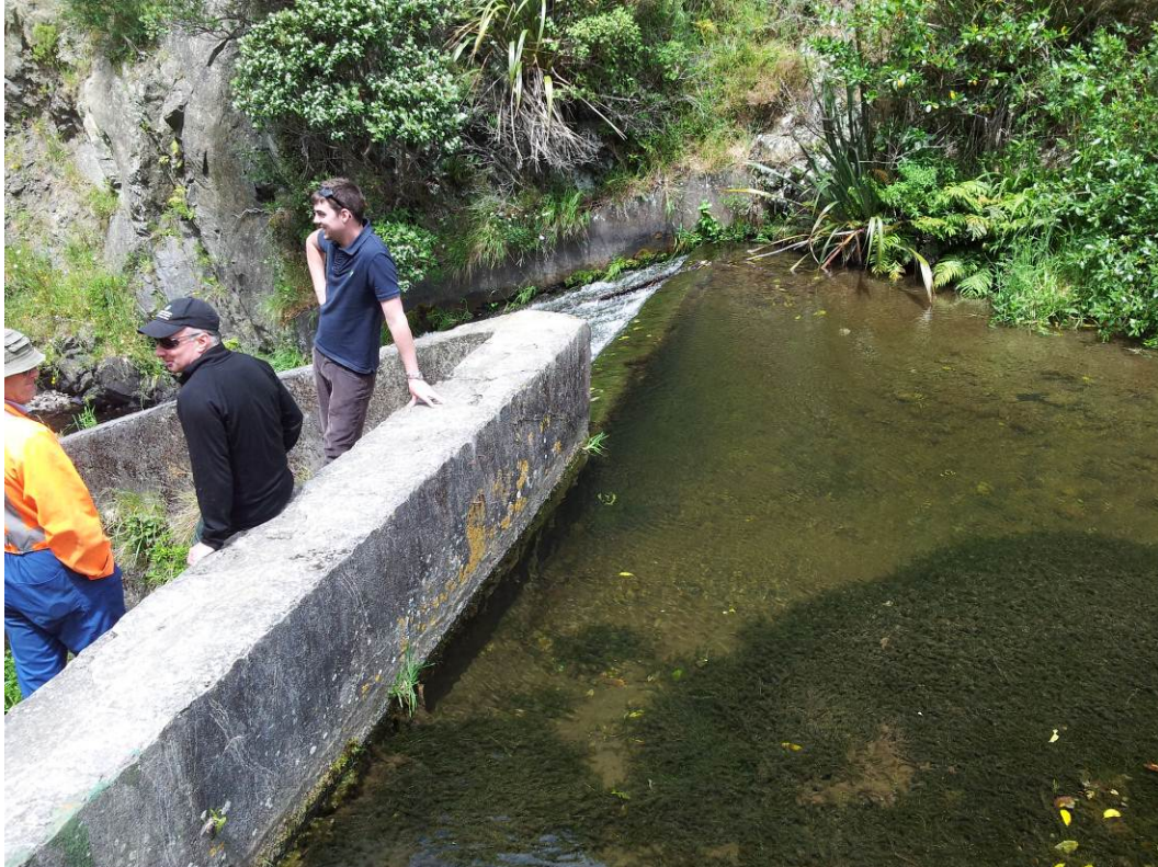
Photo 14: Woollen Mills dam upstream face, spillway crest, and right abutment. Note shallow depth to impounded gravels (less than 0.5m).
