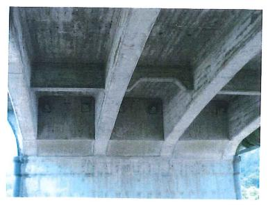
Self-compacting concrete was used to strengthen the diaphragms and abutment where the post tension bars were required and access for pouring and compacting was difficult. This was a great success and ensured the integrity of the final product in place.
