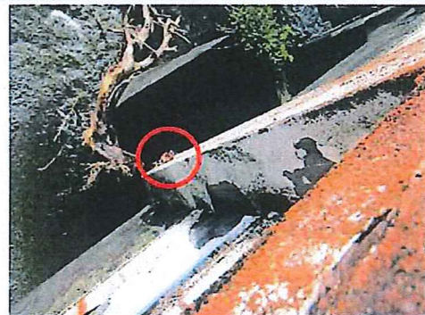
Monitor corrosion of handrail fixings - Note nut failed, no movement detected.
