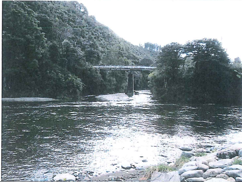
Looking upstream at bridge.
