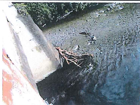
Centre pier - Note clearing of flood debris ideally should be carried out. - Review if scour resulting from the flood debris is exposing the piles of the original bridge's pier.
