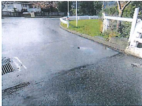
Monitor settlement of left hand approach.
