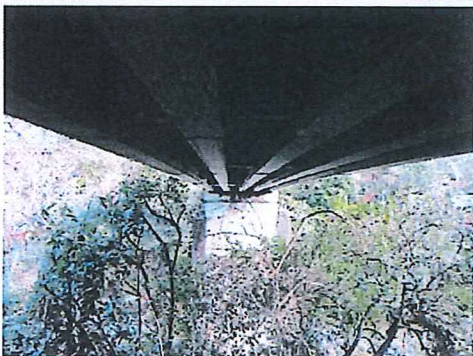
Centre pier - Note clearing of flood debris ideally should be carried out. - Review if scour resulting from the flood debris is exposing the piles of the original bridge's pier.
