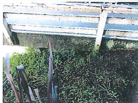
Right hand abutment - Very limited access.
