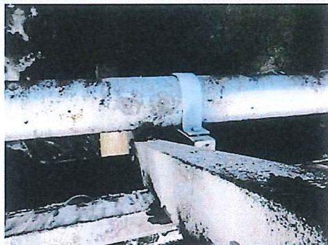
Monitor corrosion of handrail fixings - Note nut failed, no movement detected.
