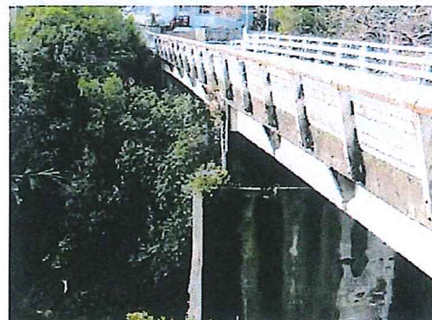
Clearing of vegetation from pier caps is an outstanding action.
