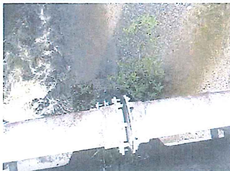
Clearing of vegetation from pier caps is an outstanding action.
