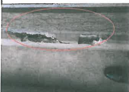
7. Location of spalling concrete in lower terrace seating
