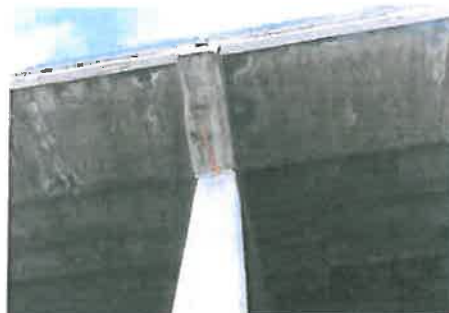
4. Location of cracks in cantilever beam
