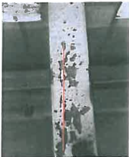
11. Location of crack along central lower floor beam
