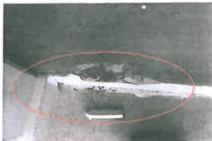
7. Location of spalling concrete in lower terrace seating
