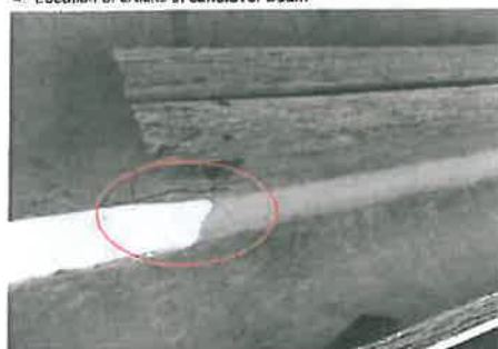
4. Location of cracks in cantilever beam
