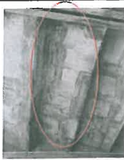
12. Location of cracks in patches under upper seating
