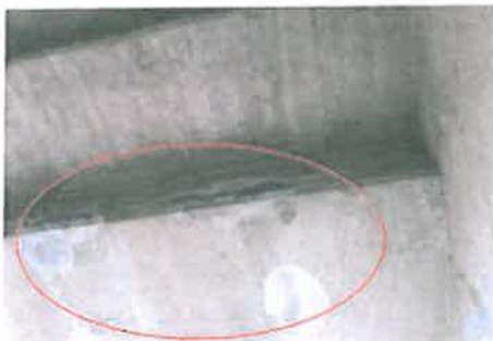
15. Location of concrete efflorescence in upperside of upper terrace seating
