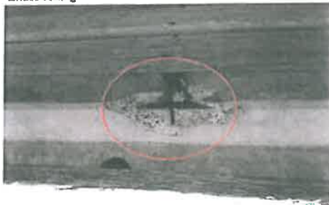
15. Location of concrete efflorescence in upperside of upper terrace seating
