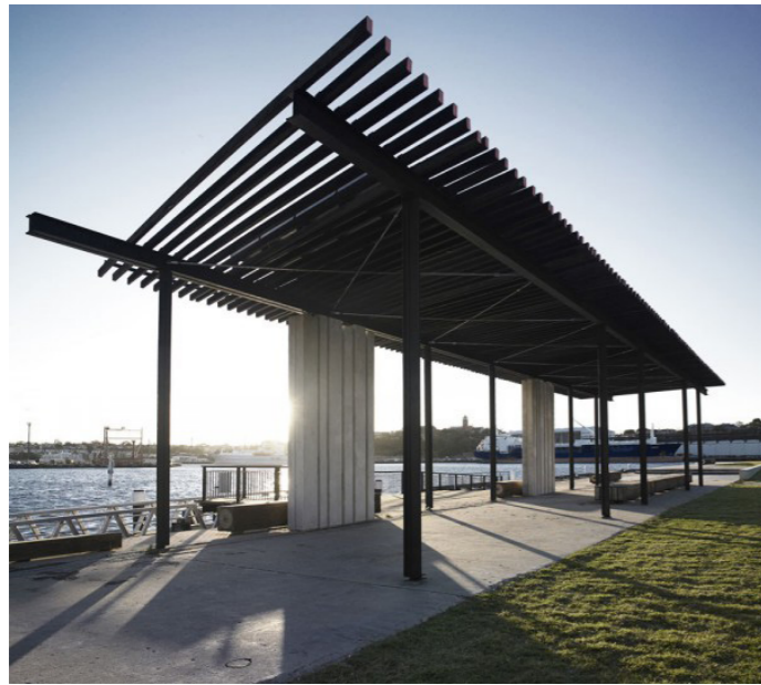
Pirrama Park - Sydney | Location - Experience and accessibility - Forms and Materials
