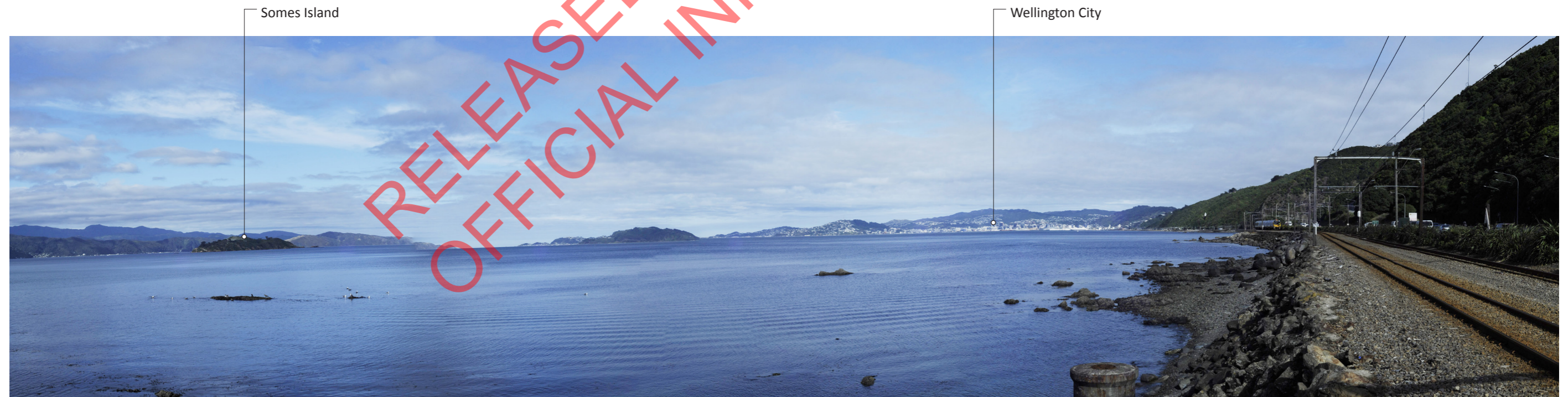
View towards Wellington City - from near possible pedestrian/cyclist shelter/station @ approximate chainage 4150.
