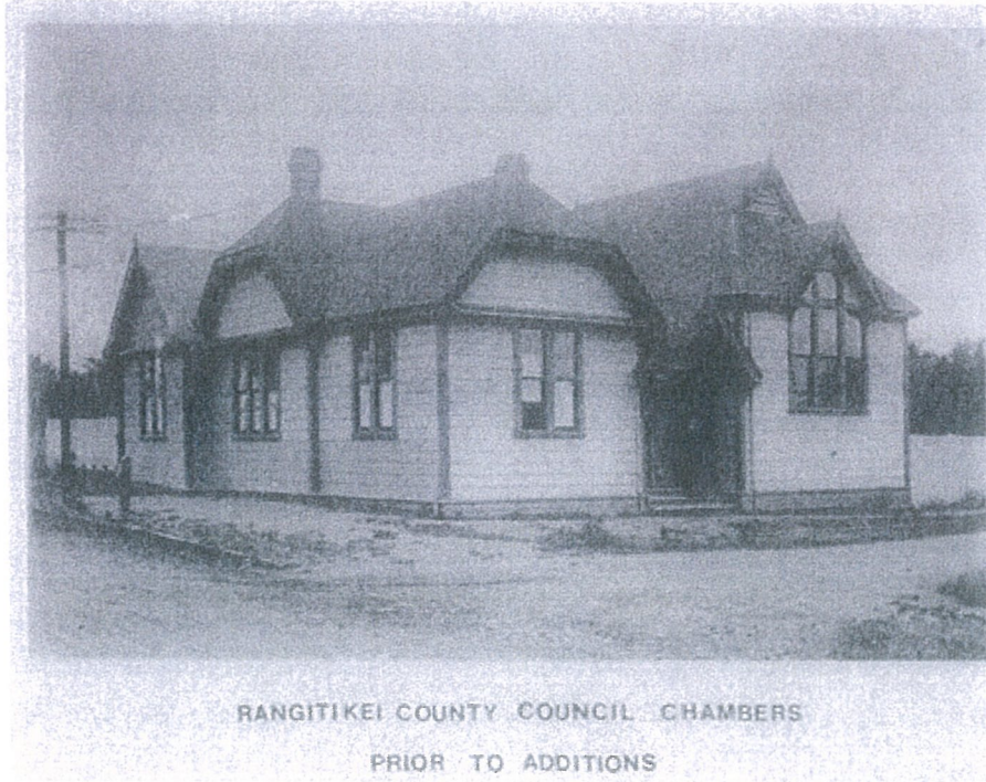
Original Building That Was Demolished 1916 - 1923
