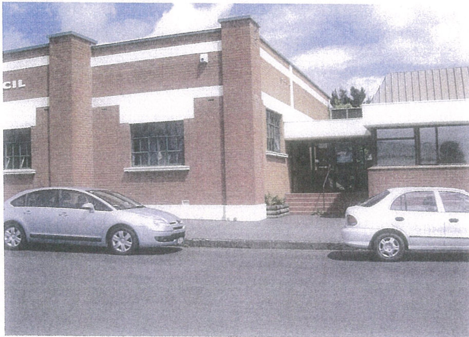
Main Council Office Building Link To Annex Building
