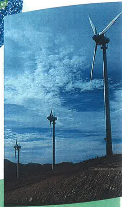
Alternative sources of energy – wind and wave power generators, with small hydroelectricity generating schemes, are seen as part of local energy solutions.
