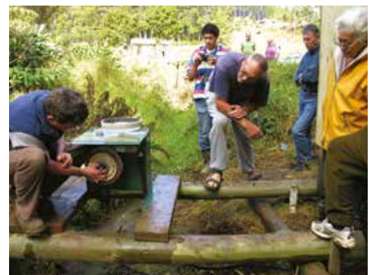
Renewable energy at Waipoua.
