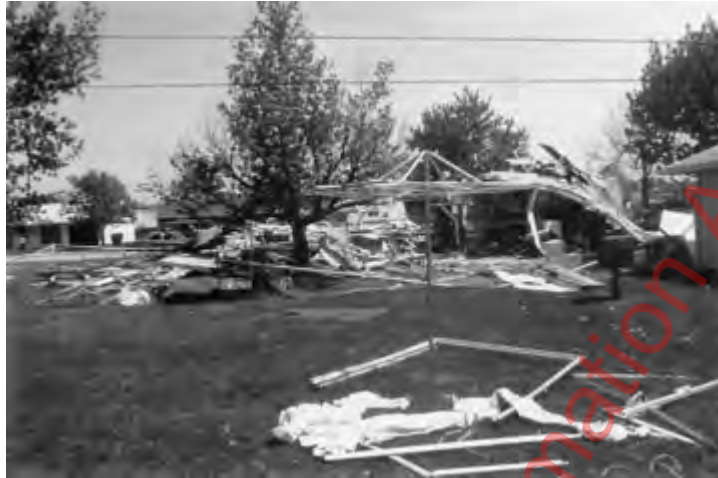
FIGURE 21.3.2 High-Order Damage Shown by Shattered and Splintered Remains of a Four-Bedroom House.
