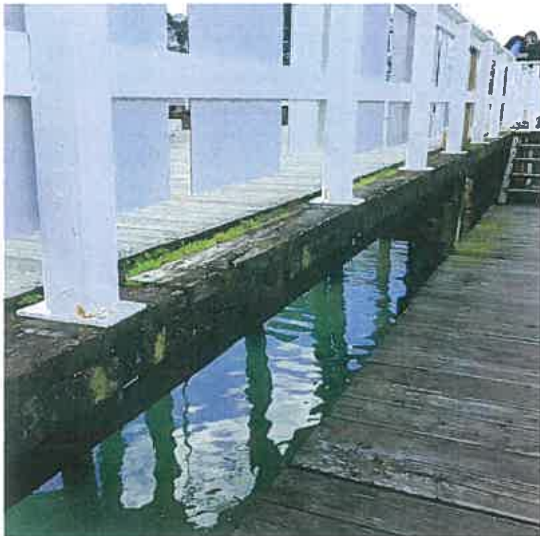
Outer boundary timber planks on approach bridge started rotting that requires cleaning and renewal and also requires renewal of handrail post footing plate
