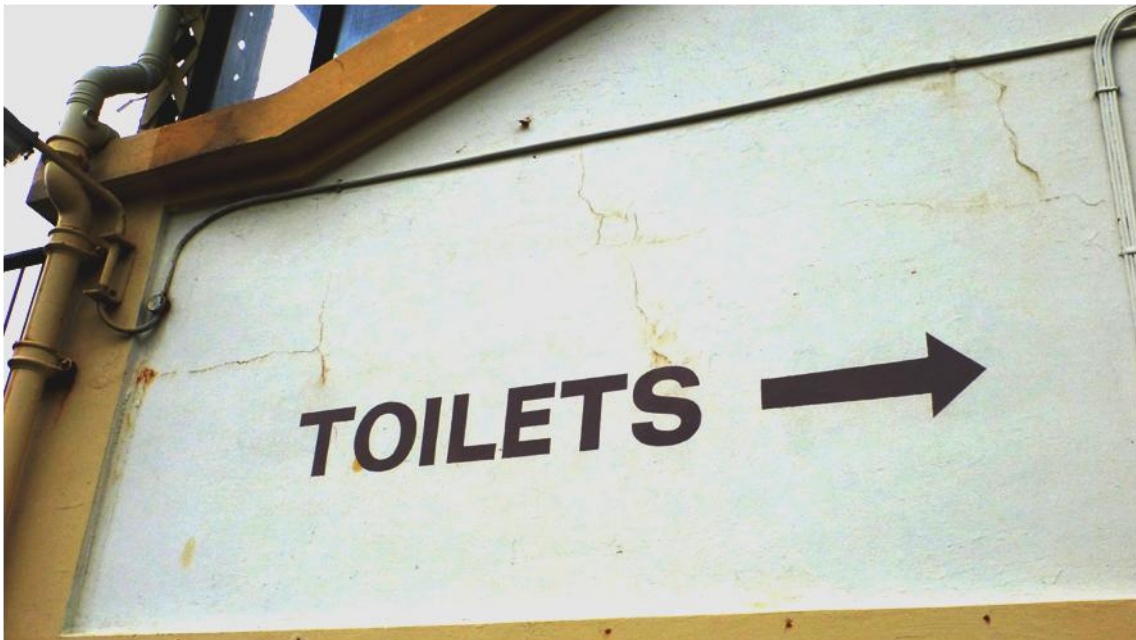
Figure 9. Cracking in the solid plaster finish applied to the northern elevation.
