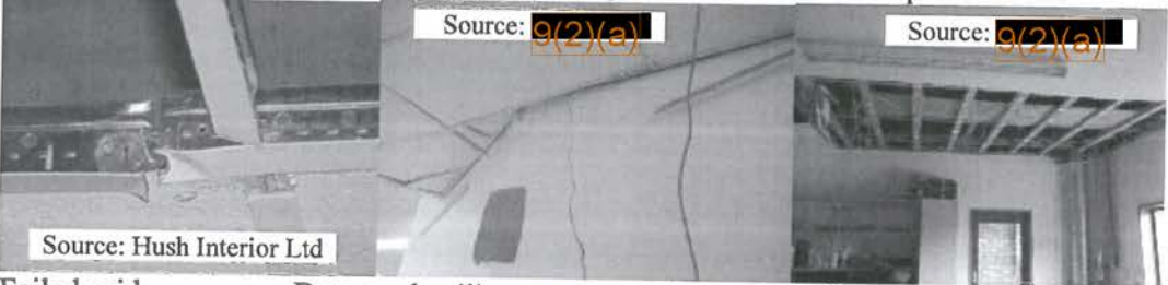
Collapsed plasterboard
