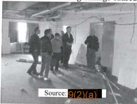
Damaged ceiling being cleared
