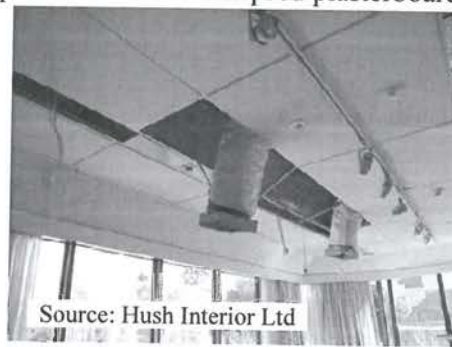
Ceiling damage caused by interaction with service
