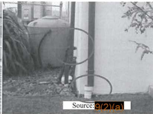
Tank rolled over an electrical unit on the roof Detached pipes due to building movement
