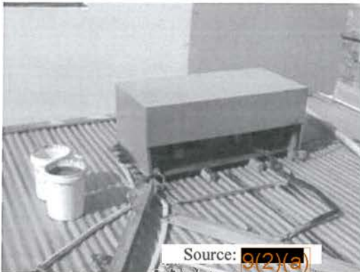
Tank rolled over an electrical unit on the roof Detached pipes due to building movement
