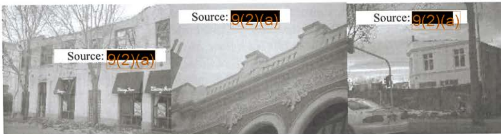
Parapet damage/collapse
