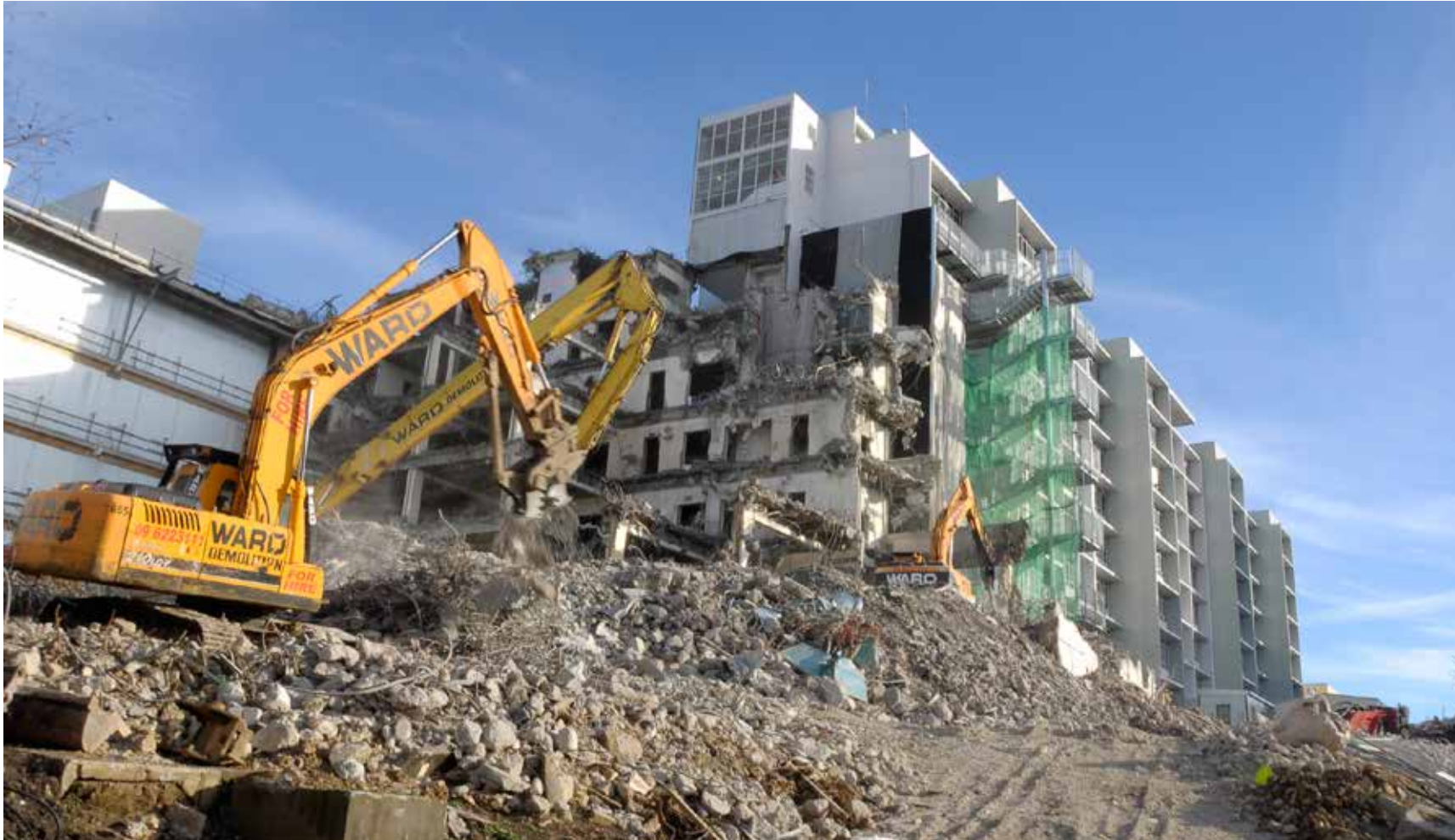
Demolition of the Smith building
