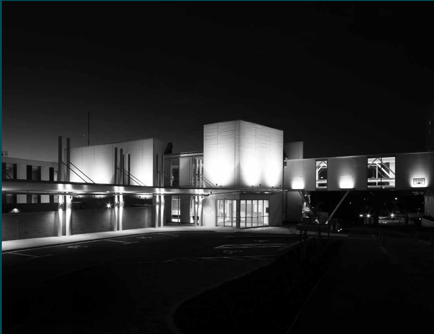
New Older Persons and Rehabilitation Building, Hamilton
