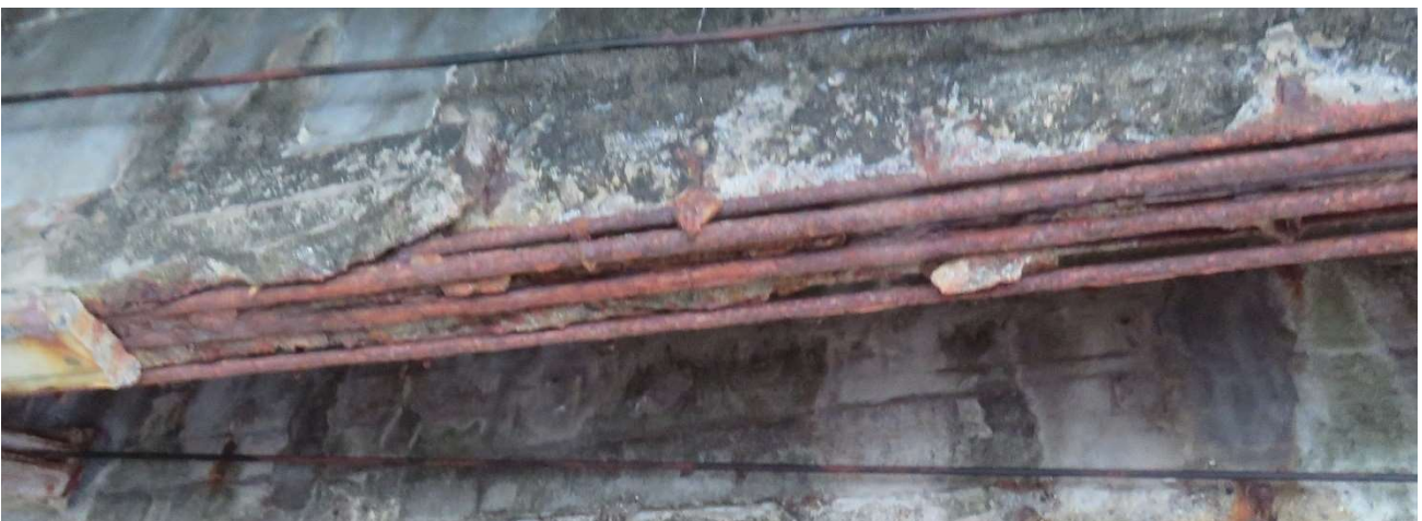
Photo 3 – Beam soffit – Span 5
