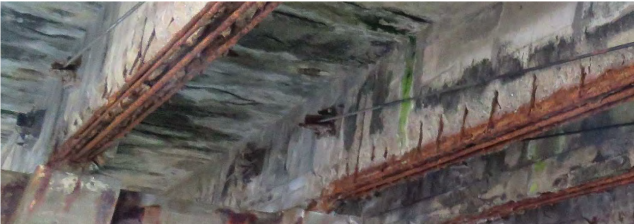
Photo 4 – Beam soffits – Span 3
