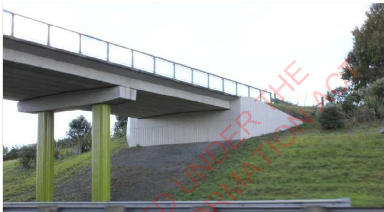
Figure 8.2: Wilks Road Overbridge
