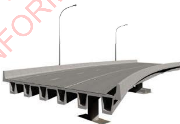
Figure 8.4: Typical Viaduct Formation
