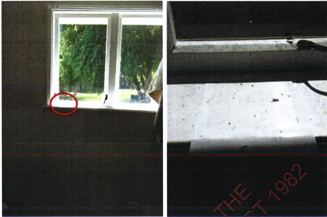
Bedroom 2 window sill: methamphetamine was detected on this surface at 1.36 \mu\text{g}/100\text{cm}^2 .
