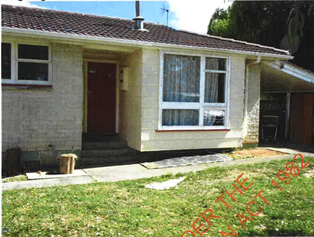
s 9(2)(a) West Harbour, view from front of property.
