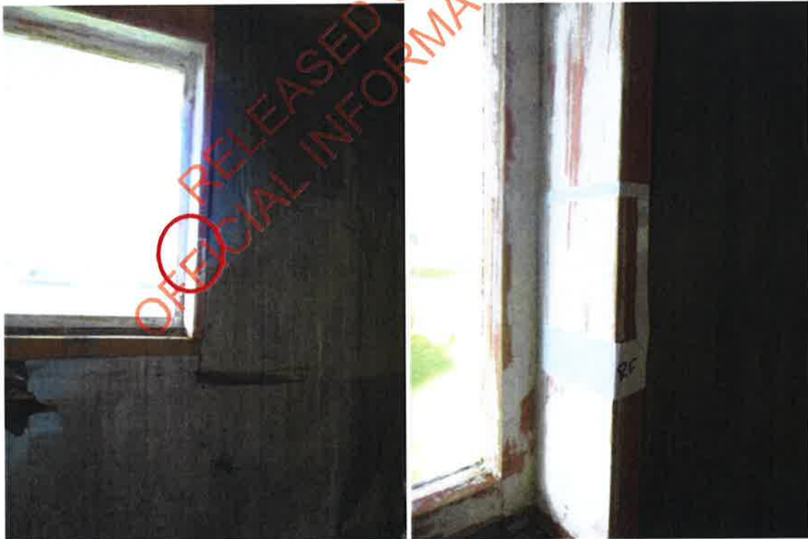
Kitchen window surrounds: methamphetamine was detected on this surface at 0.10 \mu\text{g}/100\text{cm}^2 .
